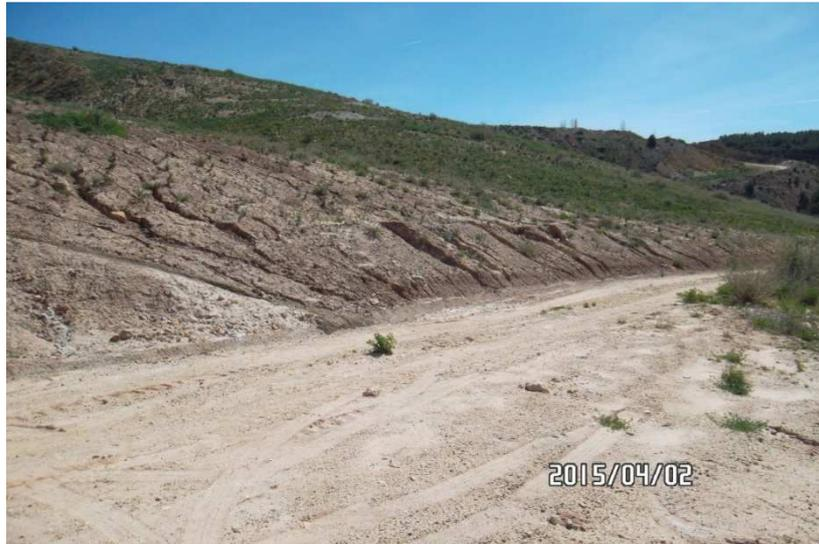
**Figure (43). Erosion on slopes and restoration accesses. Municipal District of Higuera, Valencia.**
