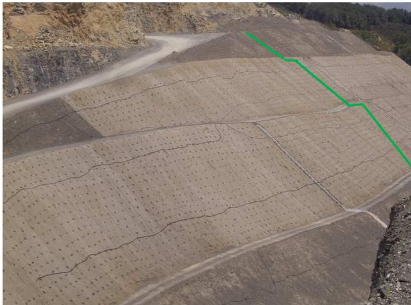
**Figure (27).** Restoration in terraces on highly sloped small surfaces, by filling with mine's own sterile material, to reduce visual impact on the A23 Highway. Municipal District of Jérica, Castellón.
