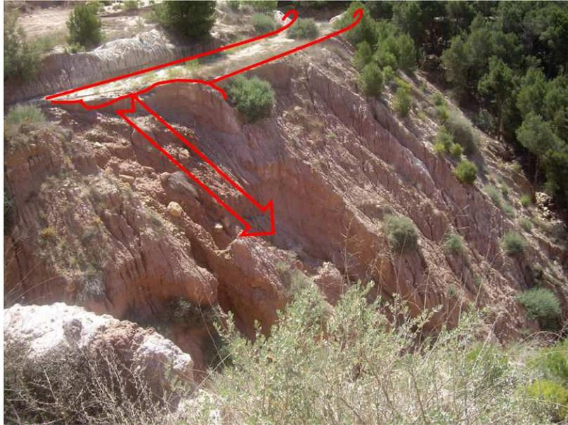
**Figure (24).** Failure of local road that connects forest public areas, due to the hydrological impact on the clayey material. Municipal District of Higuieruelas, Valencia.
