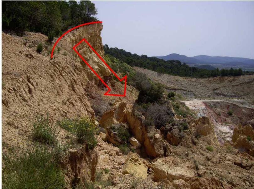
**Figure (42). Instability and landslide in red clay mines. Municipal District of Andilla, Valencia.**
