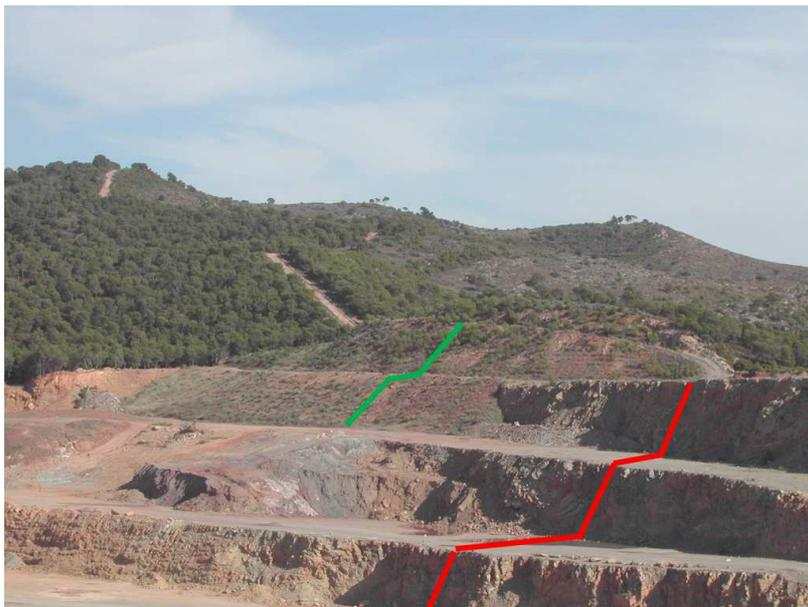
**Figure (29). Restoration of slope-berm profile after operation of the mine with same configuration. Municipal District of Sagunto, Valencia.**
