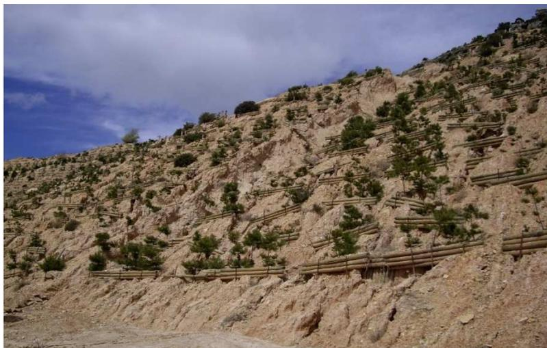
**Figure (53).** Fascines have failed to stop the erosion of the slope. Municipal District Alpuente, Valencia.
