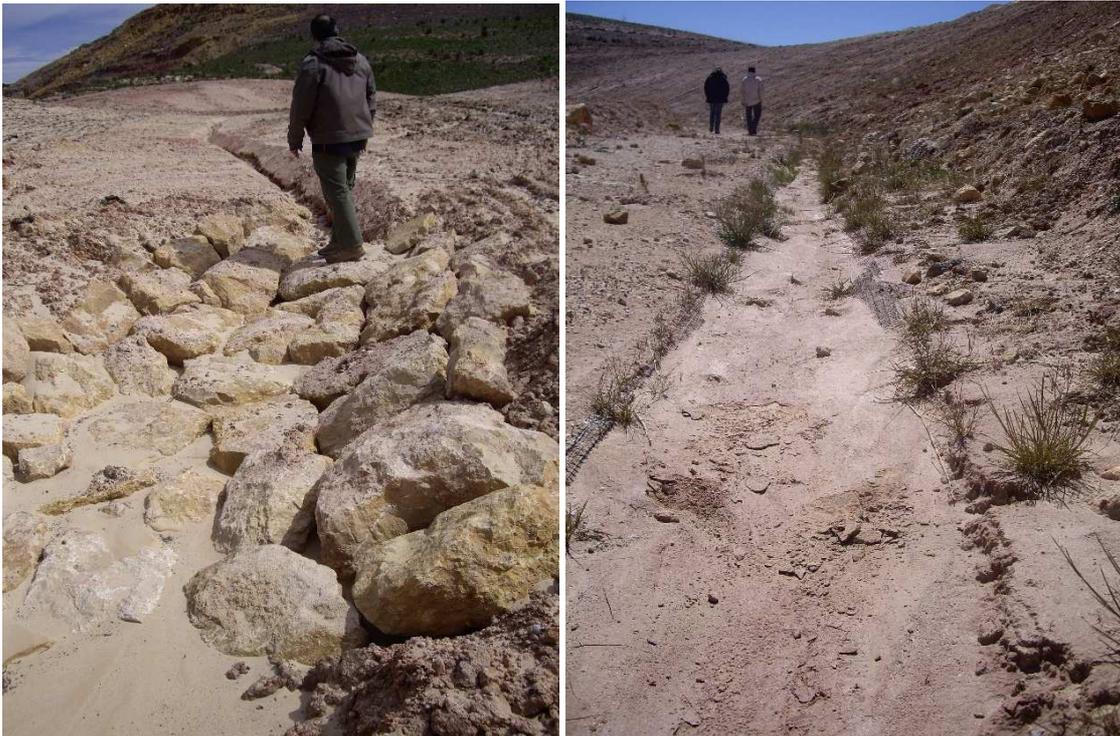
**Figure (25).** Stone banks and ditch sedimentation and after restoration. Municipal District of Higuieruelas, Valencia.
