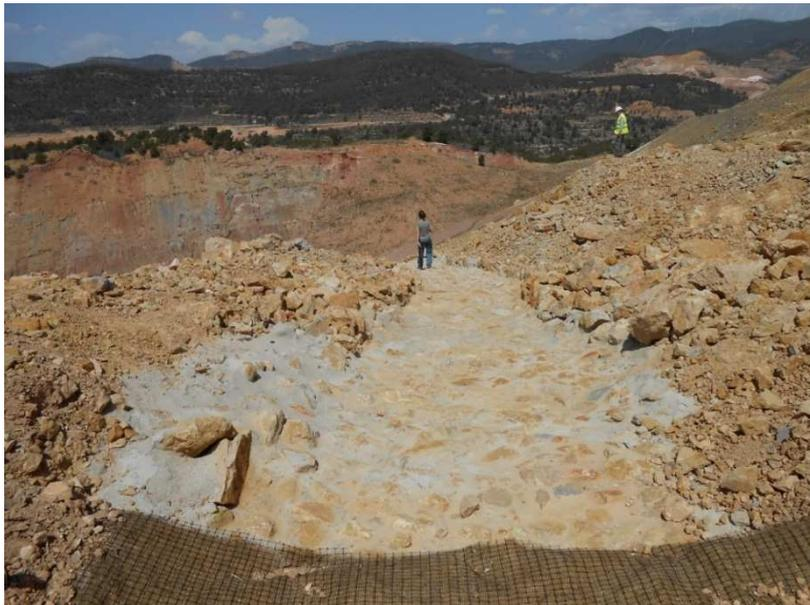
**Figure (33). Concrete and limestone channels in clay mine. Municipal District of Higuera, Valencia.**
