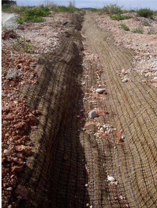
**Figure (38).** Trench with vegetable net placed as soon as the restoration is completed. Municipal District Higuera, Valencia.
