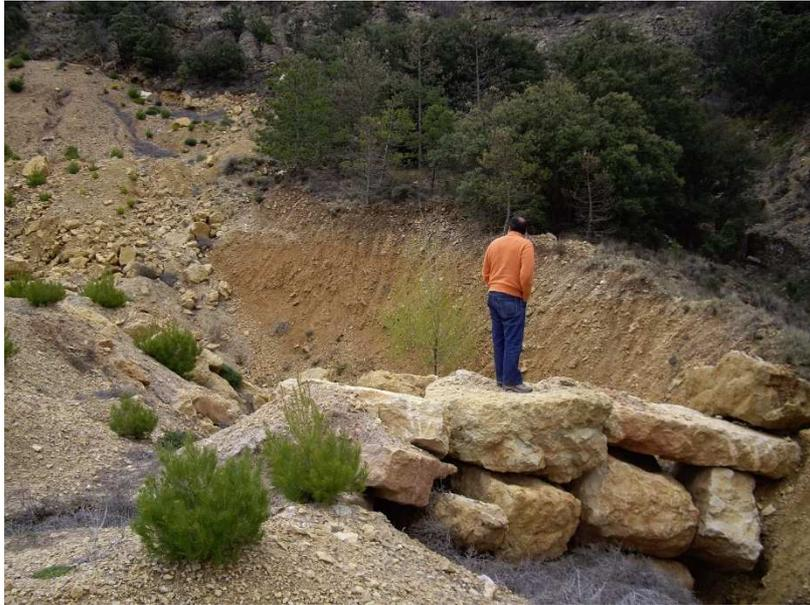
**Figure (34). Rip-rap for retention of eroded limestone. Municipal District of Alpuente-Aras, Valencia.**
