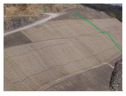
Figure (27). Restoration in terraces on highly sloped small surfaces, by filling with mine's own sterile material, to reduce visual impact on the A23 Highway. Municipal District of Jérica, Castellón.
