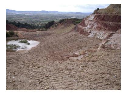
Figure (48). Slopes and water impoundment. Seven (7) years after restoration works there is no vegetation. Municipal District of Losa del Obispo, Valencia.
