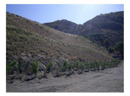
Figure (58). Drip irrigation of vegetation at toe of the slope. Municipal District Alicante, Alicante.
