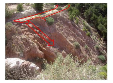
Figure (24). Failure of local road that connects forest public areas, due to the hydrological impact on the clayey material. Municipal District of Higueruelas, Valencia.
