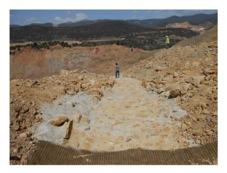
Figure (33). Concrete and limestone channels in clay mine. Municipal District of Higueruelas, Valencia.
