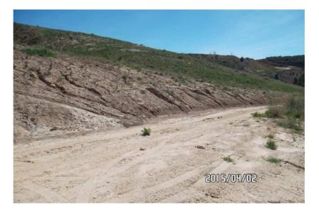
Figure (43). Erosion on slopes and restoration accesses. Municipal District of Higueruelas, Valencia.
