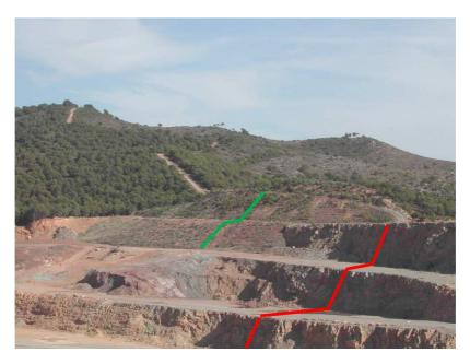
Figure (29). Restoration of slope-berm profile after operation of the mine with same configuration. Municipal District of Sagunto, Valencia.
