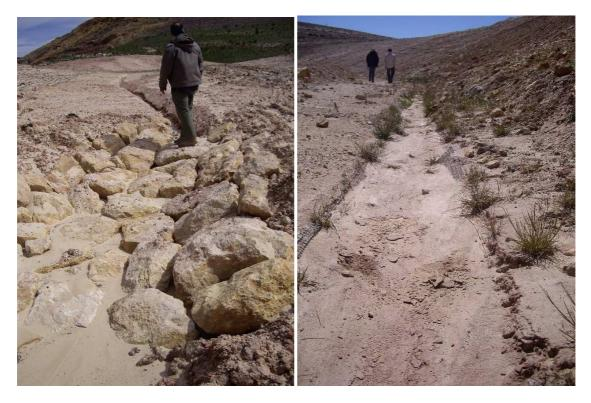
Figure (25). Stone banks and ditch sedimentation and after restoration. Municipal District of Higueruelas, Valencia.
