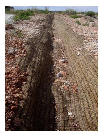
Figure (38). Trench with vegetable net placed as soon as the restoration is completed. Municipal District Higueruelas, Valencia.
